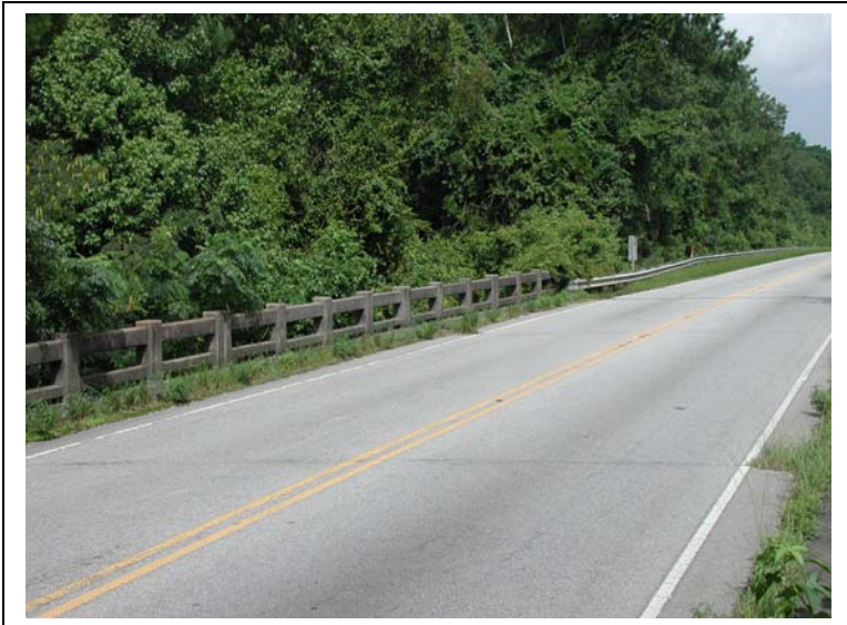
Bridge over abandoned railroad
