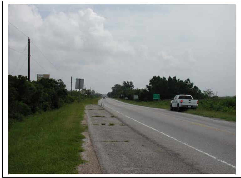
Looking North on US 17
