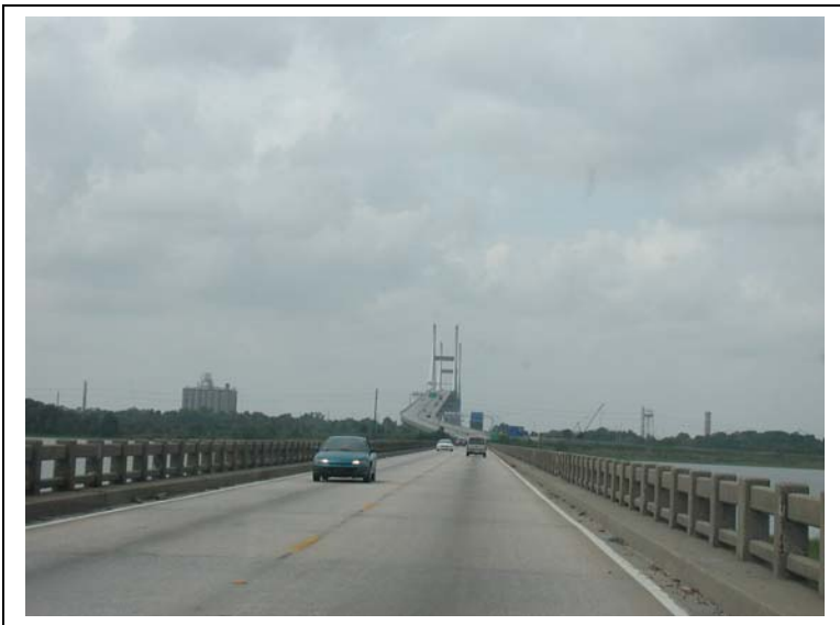
US 17 Bridge over Back River
